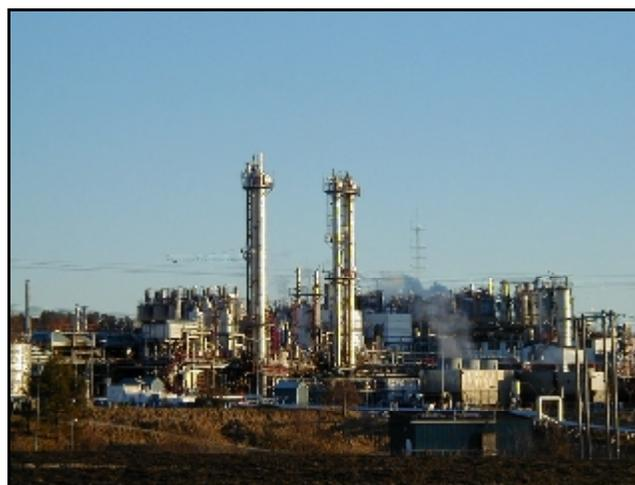
Fig. 3. Image of the polyethene plant taken from the same position as the flare measurements. The high pressure reactor is seen behind the gas purification site in the middle of the image.
