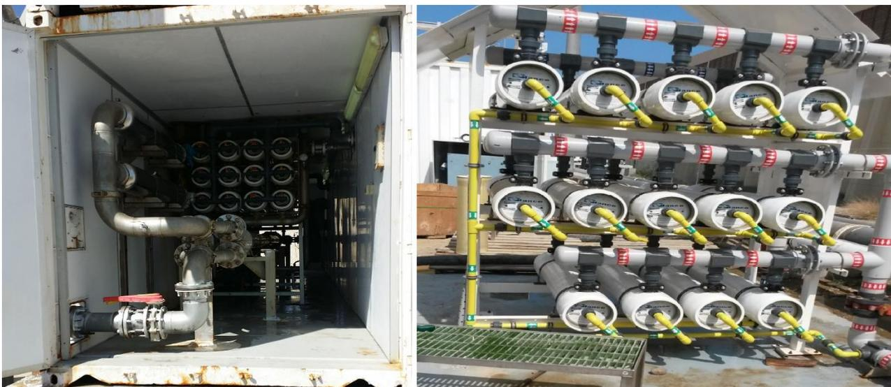
Fig. 4. Mobile system container RO desalination plant (photo: Bashitialshaer, 2015 [30]).
